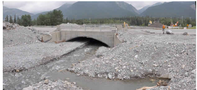
Figure 16. Downstream view of the Highway 1A bridge spanning Exshaw Creek. July 2013.
