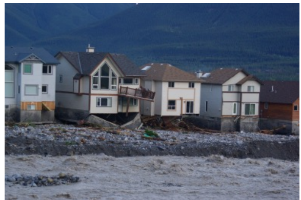
Figure 8. Damage to homes along left (east) bank of Cougar Creek between Elk Run Boulevard and Highway 1.
