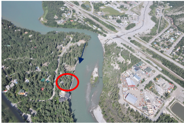
Figure 17. Aerial view of the confluence of Exshaw Creek with the Bow River. Deposition at the mouth of Exshaw Creek concentrated flows along the right bank of the Bow River, resulting in bank erosion and undermining of one home (circled in red). All homes of Lac des Arcs are located on Heart Creek fan.
